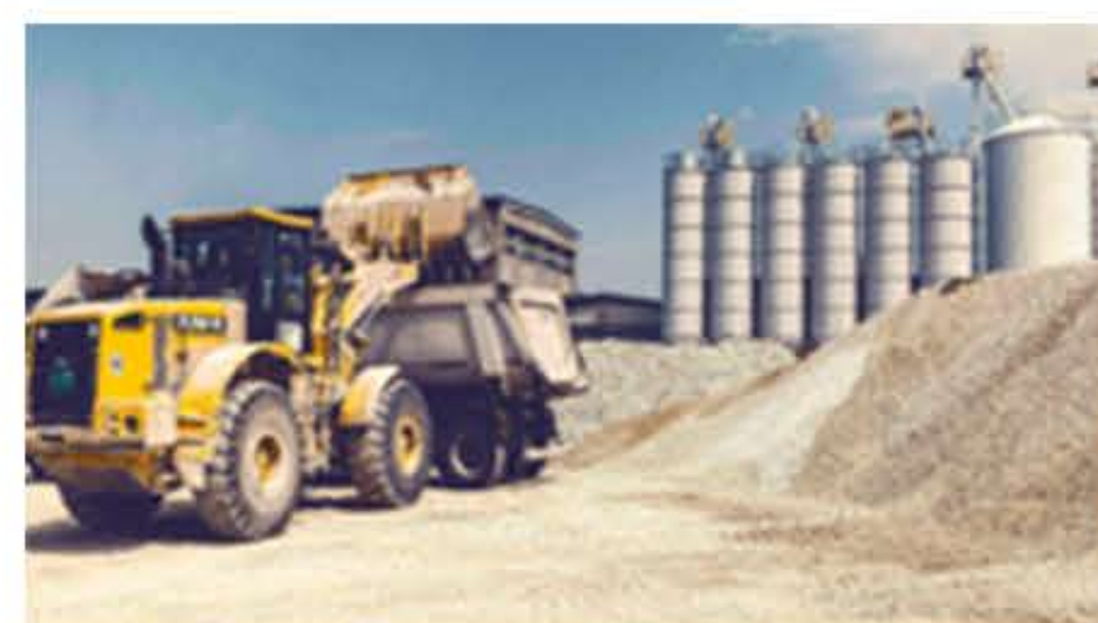
Run Hours Monitoring
